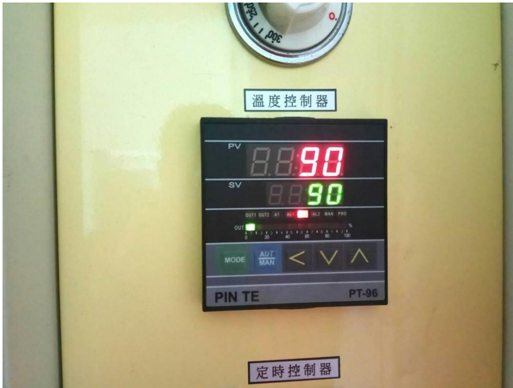
Heat conditioning -II
