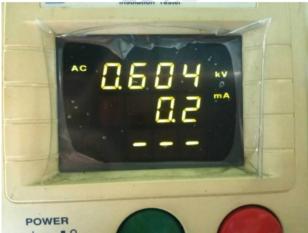
Leakage current test -II
