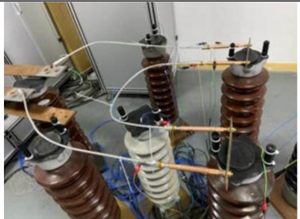
Temperature rise tests
