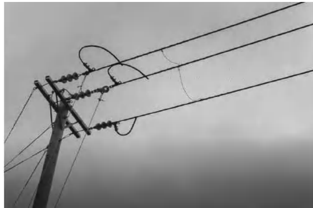
I. Three-phase overhead lines with cable support installed.
