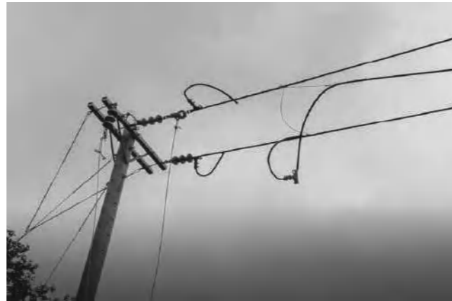
II. Chardon Cable Support Rope mounted onto a downed cable.
