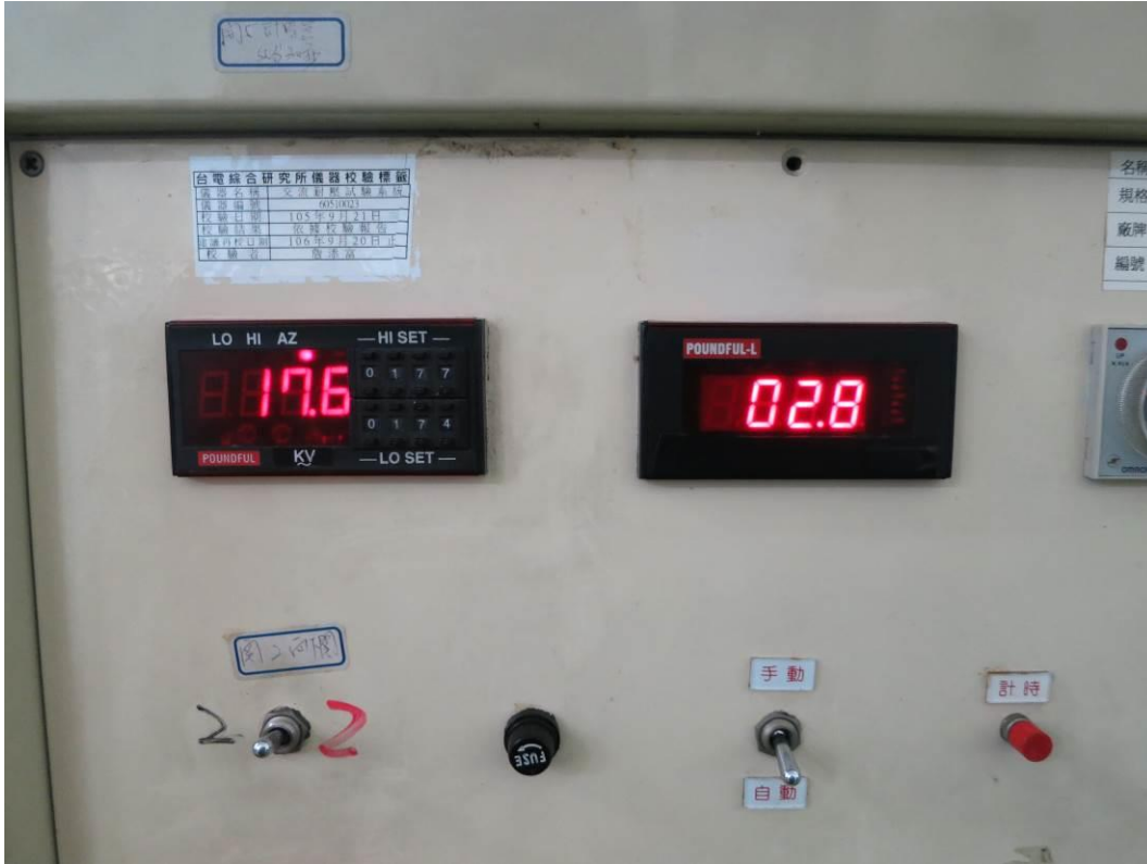
Leak Test in Progress
