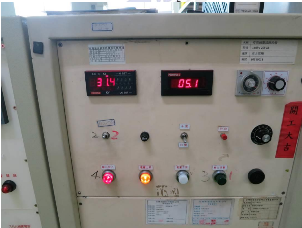
AC Withstand Voltage Testing in Progress
