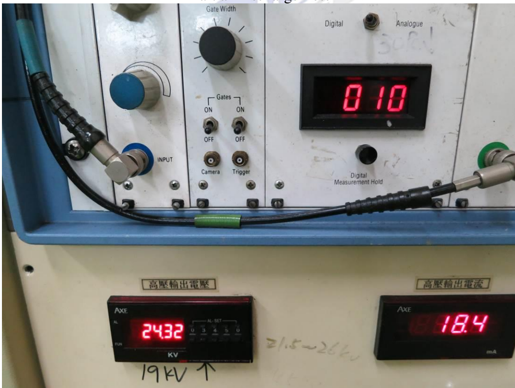
Partial Discharge Testing in Progress
