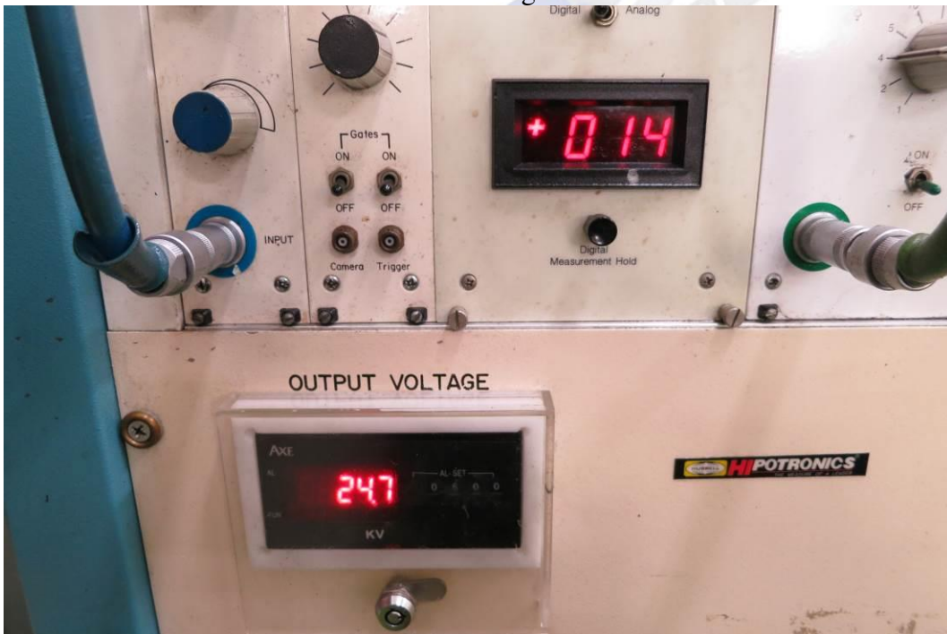
Partial Discharge Testing in Progress
