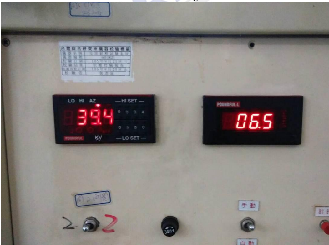
AC Withstand Voltage Testing in Progress
