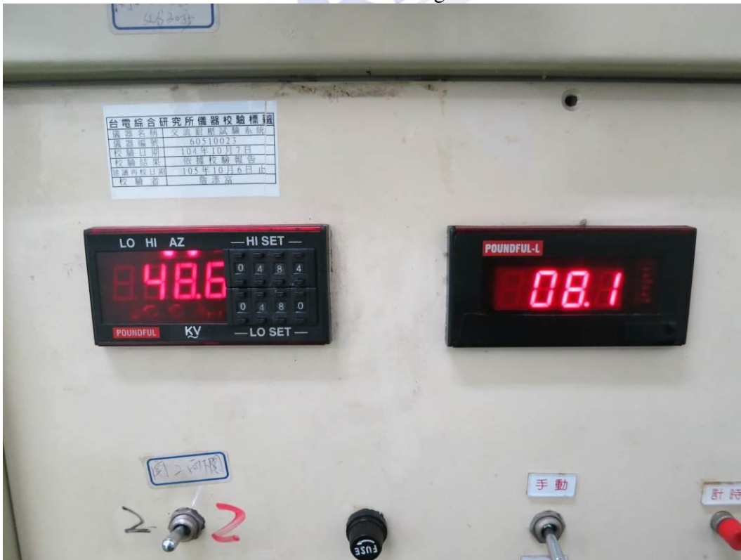
AC Withstand Voltage Testing in Progress
