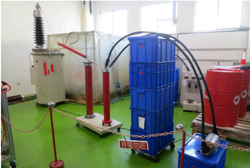
Testing Setup of DC Voltage Dry
