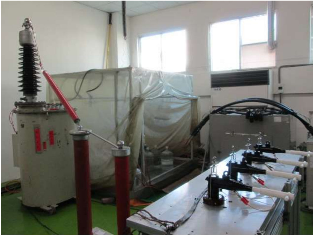
Fig 3-1 DC Withstand Voltage Test Setup
