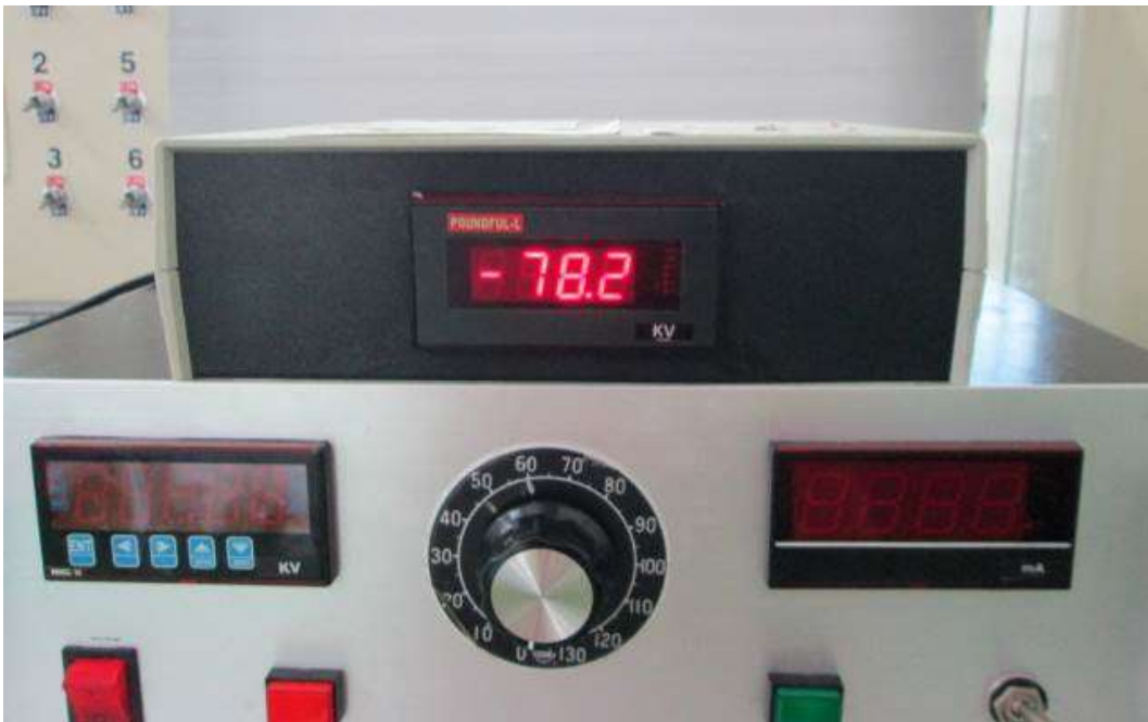
Fig 3-2 DC Withstand Voltage Test in Progress
