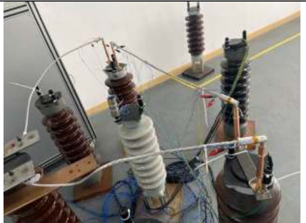
Temperature rise tests
